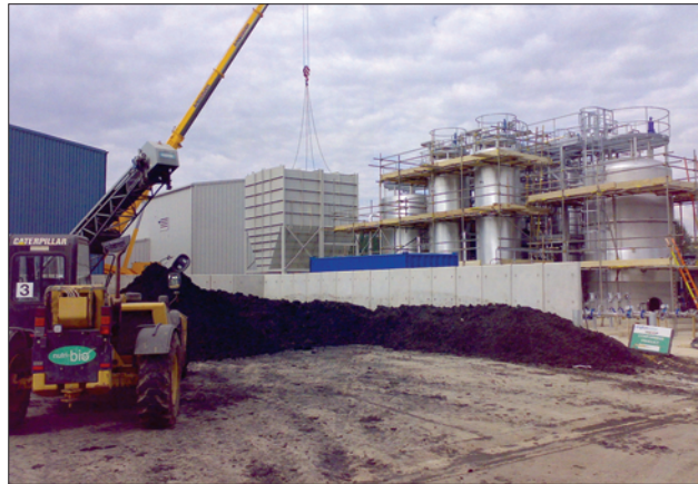
The sludge hopper is added to the processing facility
